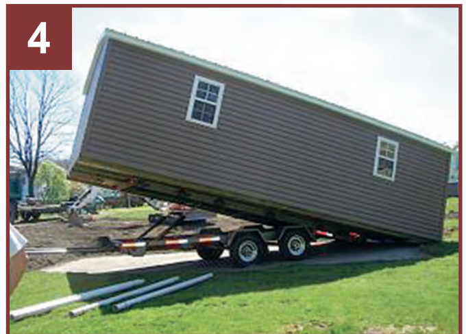
4 Shed is delivered and placed.
