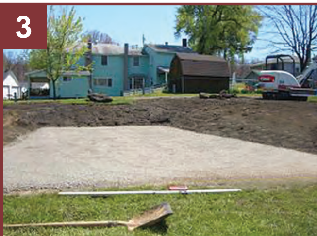
3 Approximately 4" of stone is added and compacted.
