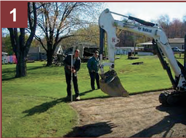
1 Check grade difference with laser transit and remove sod.
